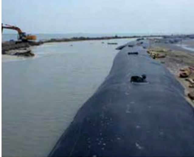
Figure 3-34: Cofferdam of Geotextile Tube
