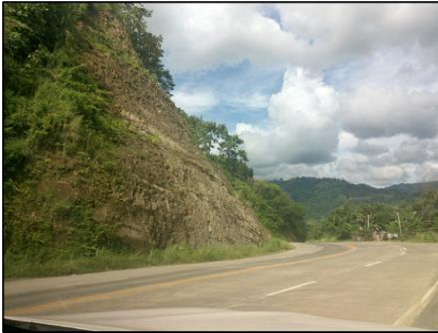
Plate 4-12. Beddings that are Daylighting with Respect to the Orientation of the Roadcut in KM 1592
