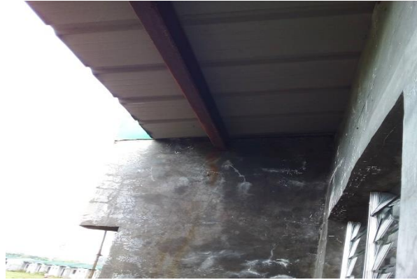
Roof with Reported Leakage
