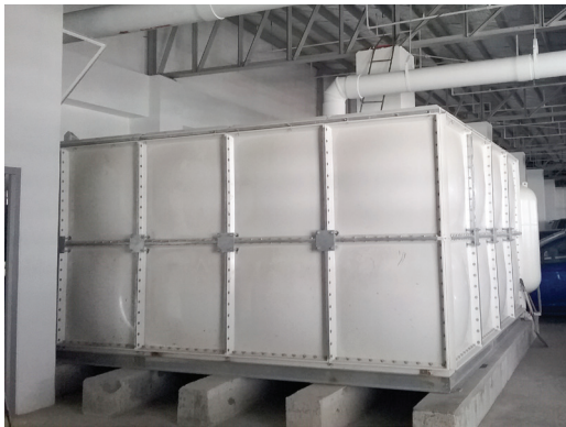
FIGURE 77: Modular type storage tank for rainwater collection directly beneath roof area. Rainwater collecting tank is fed directly via downspouts from roof gutter.
