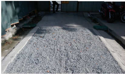
Gravel bed on construction site to help scrape-off dirt from vehicular tires before entering public street
