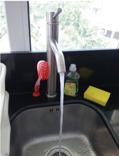
FIGURE 69. Water efficient kitchen tap with aerator
