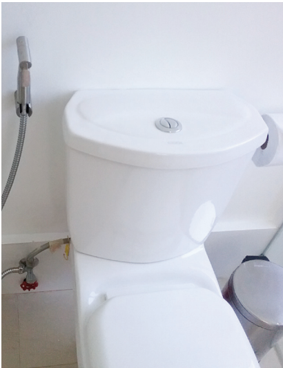
FIGURE 72. Water efficient water closet with dual-flush and water efficient hand spray bidet
