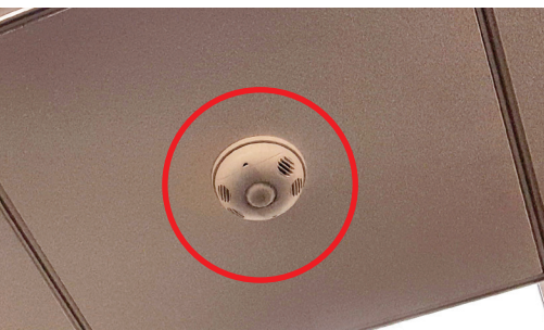
FIGURE 56: An occupancy sensor mounted on the ceiling of a conference room
