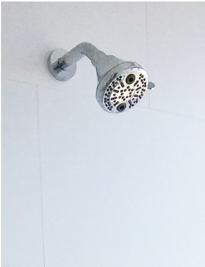
FIGURE 71. Shower head with adjustable water spray
