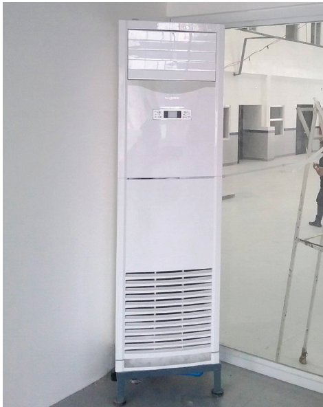
DIRECT EXPANSION (DX) – air-conditioning system uses refrigerants as cooling medium. This system includes energy efficient systems such as the variable refrigerant flow (VRF) and inverter type air-con units.
