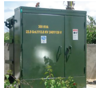
FIGURE 63: A three phase dry-type transformer
