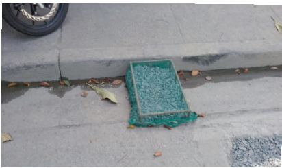
For sediment filtering at drainage way
