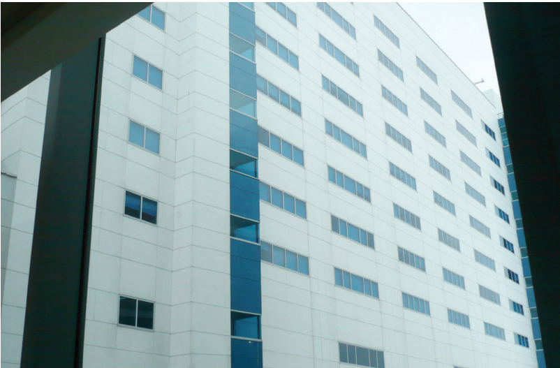
FIGURE 16: Concrete wall in paint finish with moisture barrier properties
