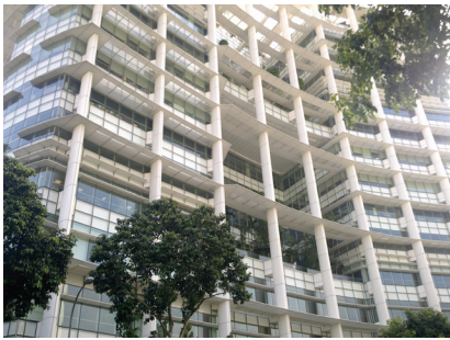
FIGURE 20: Completed building showing the application of sun breakers over the windows
