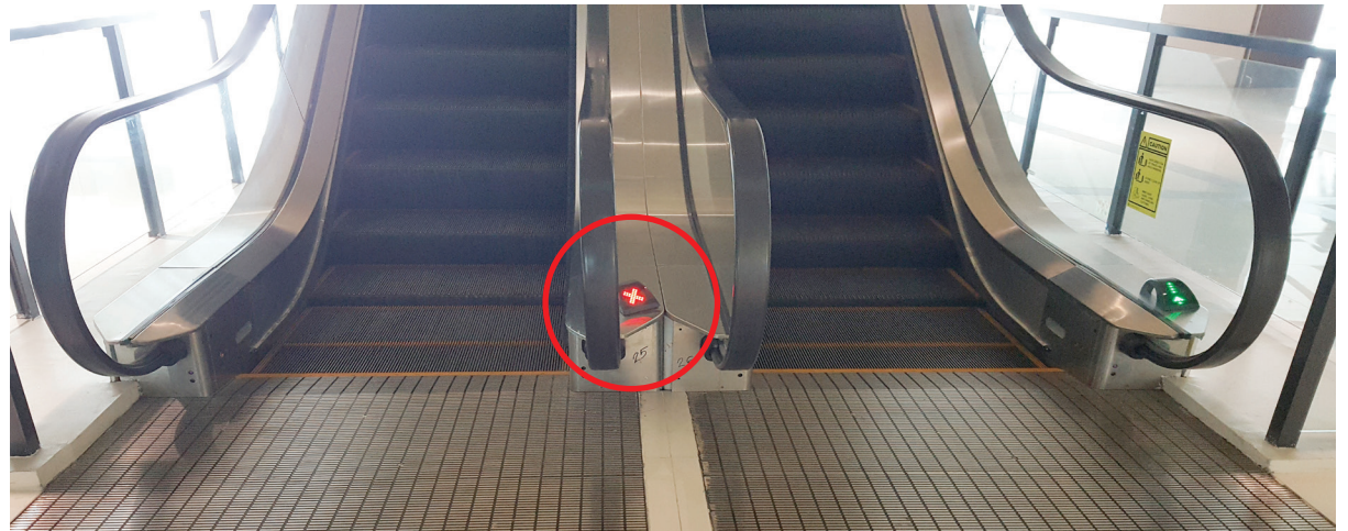
FIGURE 59: Escalator showing the placement of sensors used to detect passengers
