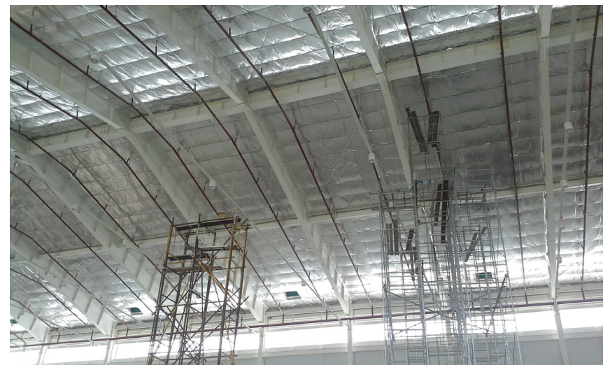
FIGURE 34: Mineral wool insulation installed under metal roof
