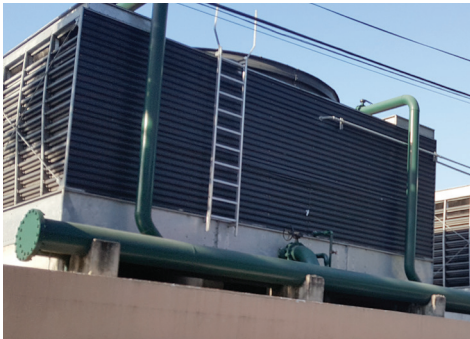
WATER-COOLED CHILLED WATER COOLING SYSTEM – employs water as the condensing medium and uses pumps to circulate the water through the condenser and out to a cooling tower that ejects the heat to the atmosphere.
