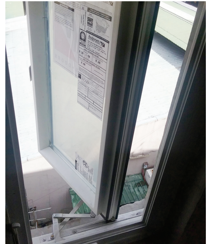
FIGURE 8: Window frame fully sealed with gasket and weather stripping all around.
