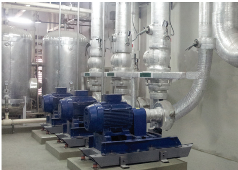
PUMPS – help circulate water within the chilled water system
