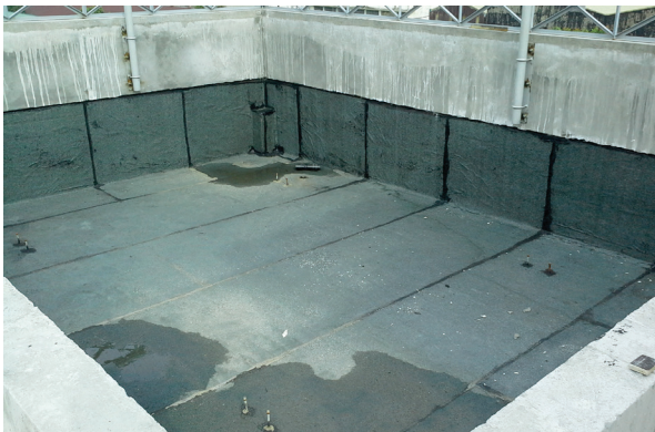
FIGURE 18: Roofdeck sealed with waterproofing membrane
