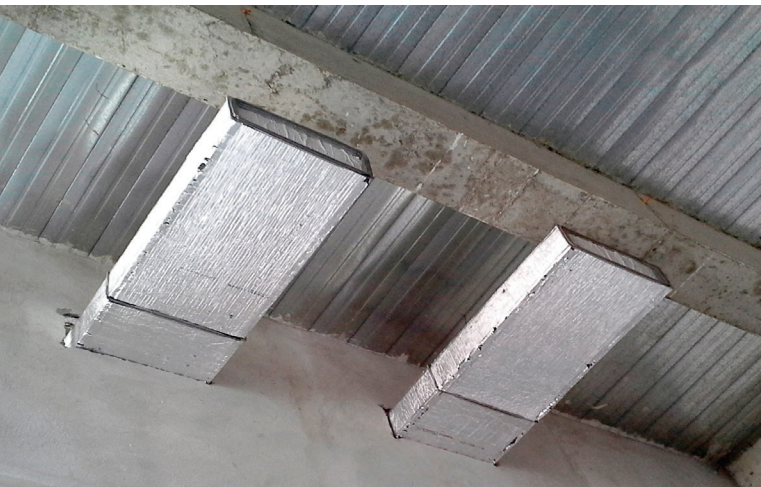
FIGURE 9: Duct penetration through wall ready to receive sealing material. This is to prevent transfer of air and moisture between spaces.
