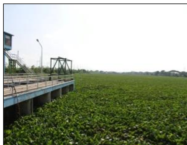
Figure 13: Labasan Pumping Station: trash trap (left) and water hyacinth accumulating in the retention pond (right)
