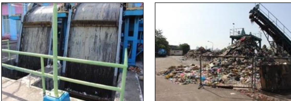
Figure 2: Solid wastes screen installed in Vitas Pump Station (left) and solid wastes collected by the trash traps (right)
