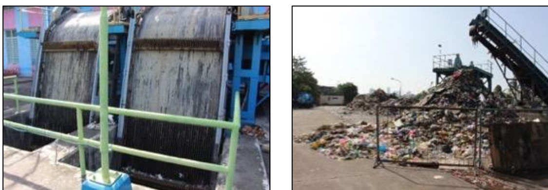
Figure 3: Solid wastes screen installed in Vitas Pump Station (left) and solid wastes collected by the trash traps (right)
