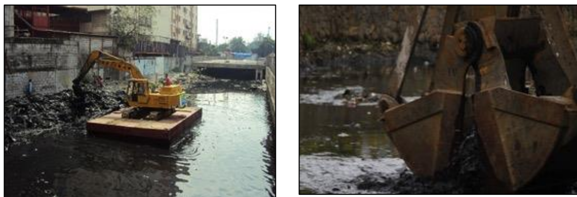
Figure 15: Dredging of narrow esteros leading to pumping stations
