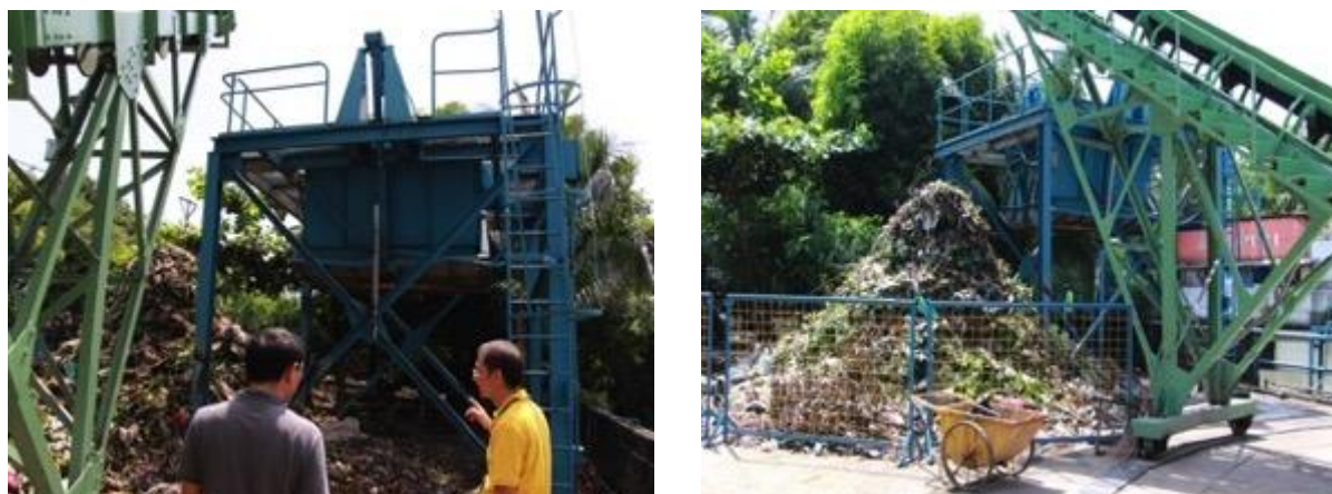
Figure 10: Solid waste collection at Paco Pumping Station
