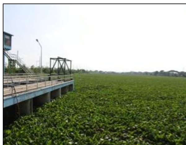
Figure 14: Labasan Pumping Station: trash trap (left) and water hyacinth accumulating in the retention pond (right)
