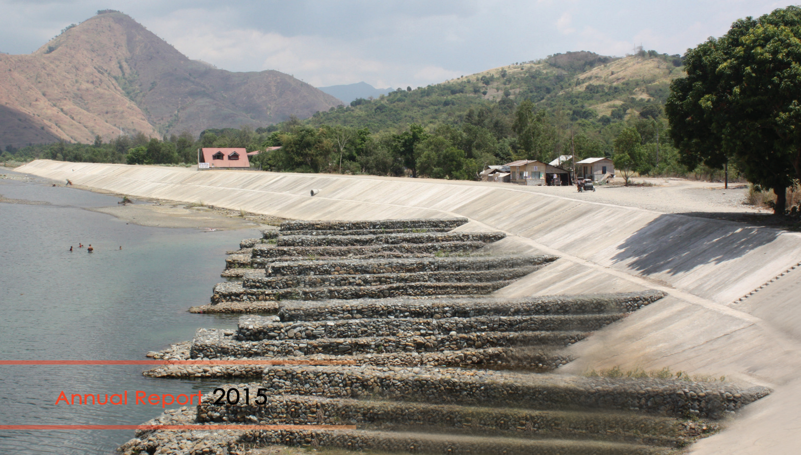
Slope protection works at Killing Dike including Tributary Dike, Cabangan, Zambales
