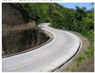
pavement (10.20 kilometers), rehabilitation of existing gravel surface, paving of shoulder with 150 mm thickness of portland concrete cement pavement along mountainous section, and improvement/rehabilitation of shoulders and drainage facilities along the existing portland concrete cement pavement for a length of 6.05 kilometers. It also includes the construction of one (1) bridge, slope protection works, masonry walls, and ancillary works. Project is 79.41% completed.
