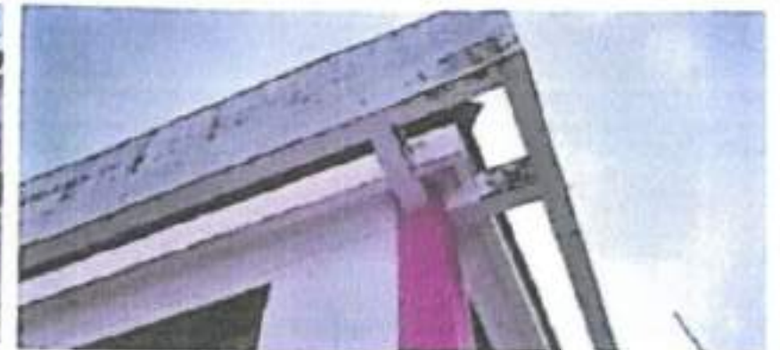
EXISTING CANTILEVER AREA
