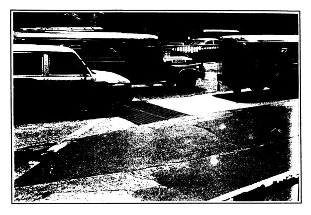
Project: Product: **DPWH – España Corner Morayta** Webdrain Sump Grates – WA655/1/P/G Consists of FB 65 x 5 mm thk spaced @ 30mm o.c. With 6mm twisted rod spaced @ 100 mm o.c. With angular frame (L75 x 75 x 9mm thk) & with I-Beam Support Hot Dipped Galvanized with BS EN ISO 1461
