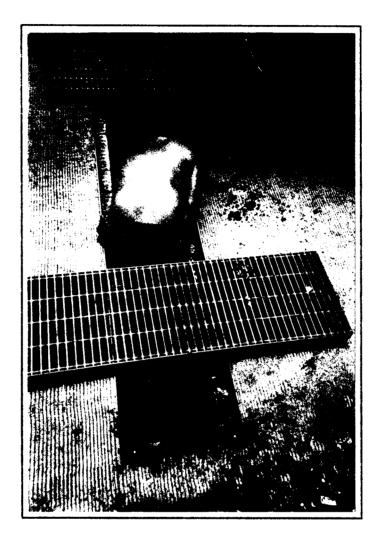
Steel grating shall be fitted in its frame by providing holding down bolts made of stainless steel or spot welded on corners and sides to provide resistance to unauthorized opening.
