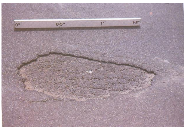
Example: Surface Failure due to delamination
