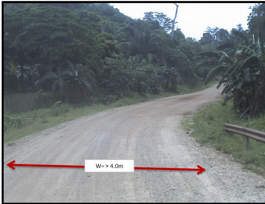
GRAVEL ROADS ( W = > 4.0\text{m} ) 2-Lanes, 2-Way, No Shoulders
