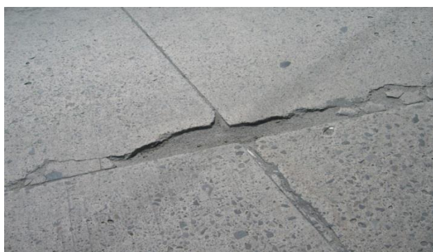
Spalling at Joints
