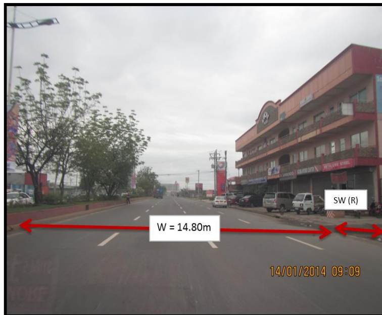
ASPHALT (W = 14.80m) 4-Lanes (with Markings), No Shoulder, with Right Sidewalk Dual Carriageway (One-Way)
