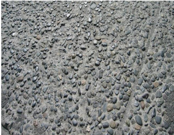
Example: Severe Scaling – rough texture
