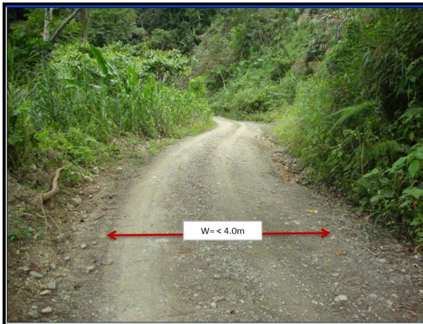
GRAVEL ROADS ( W < 4.0\text{m} ) 1-Lane, 2-Way, No Shoulders
