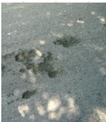
Example: Surface Failure due to wearing course deterioration
