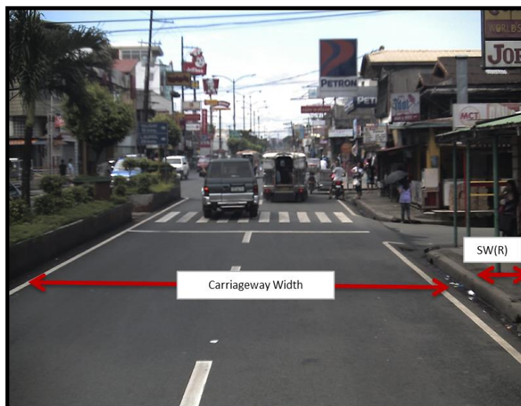
ASPHALT (W = 6.10m) 2-Lanes, 2-Way, No Shoulder on Both Sides, with Side Walk at Right Side
