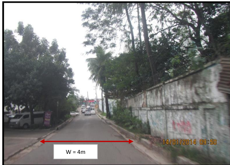
ASPHALT (W = 4m) 2-Lanes (Sub-Standard), 1-Way, without Markings, No Shoulder/Sidewalk, with Curb and Gutter
