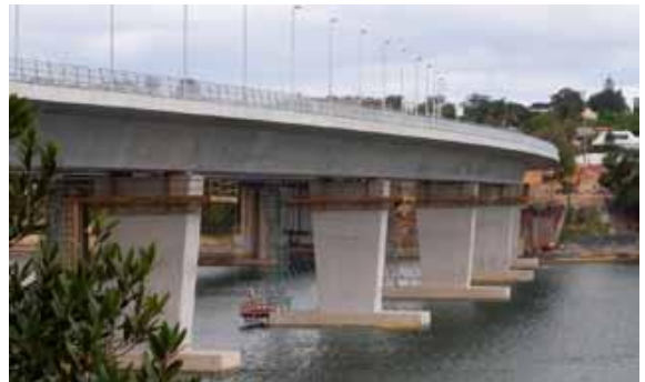
Figure 36. – Box girder in angled connection
