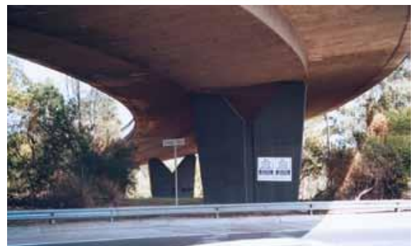
Figure 37. – Box girder in very acute angle connection
