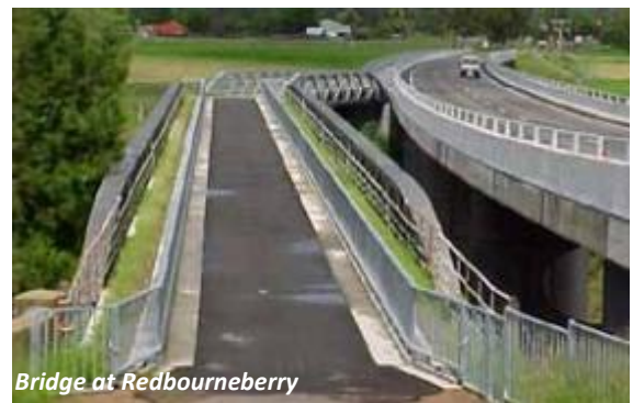
Bridge at Redbourneberry In this adaptive re-use of an old bridge, the wrought iron lattice truss bridge at Redbourneberry was duplicated and incorporated into an adjacent cycleway. The angle span at the far end was built as part of the duplication. Its design however is pastiche since it attempts to imitate the existing truss. Not only is this false and confusing but it jars with the new bypass.
