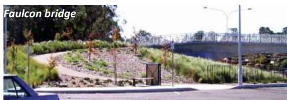
Earthworks have been utilised to cost effectively create the landscaped ramp to the Faulcon bridge over the Great Western Highway.
