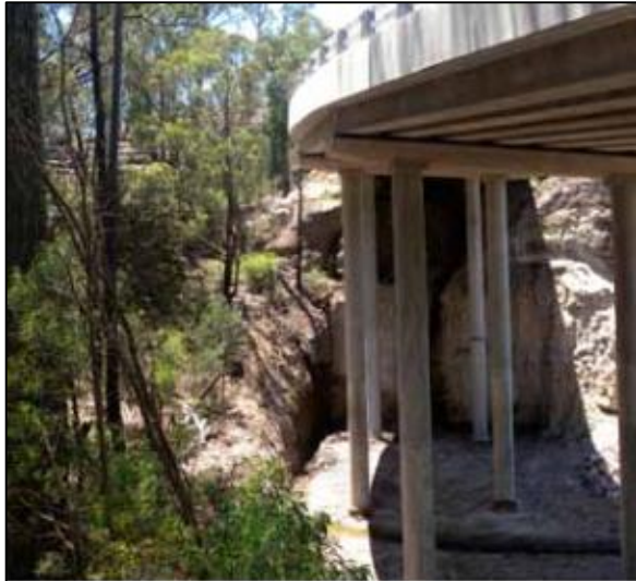
The pier widths used on this bridge next to the old wool road appear too thin and almost spindly in comparison to the depth of the girder and parapet.
