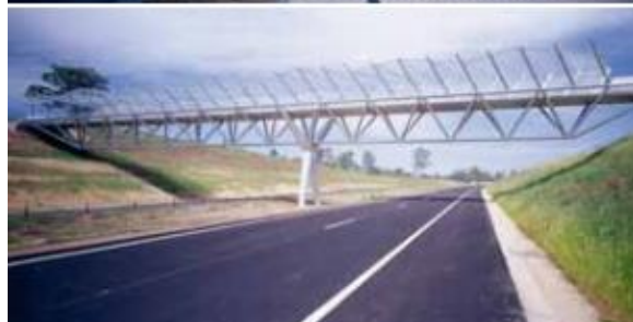
Structurally expressive form using modern materials is evident in this space-frame.
