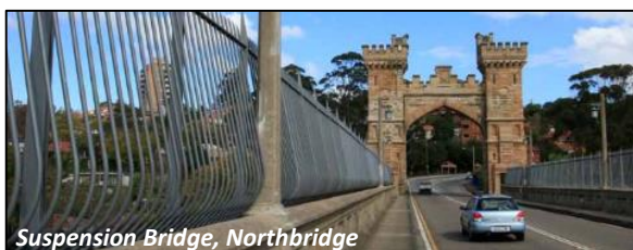
A new protective fence on suspension Bridge, Northbridge proved to be a challenging new addition to the historic structure. The style and shape of the fence was carefully considered so that it fitted with the bridge aesthetic and also prevented access over the parapets. A picket type fence proved to be most appropriate with a curved form to both add interest and make it difficult to stand on the parapet.
