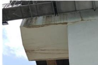
PIER 9 COPING (WATER LEAKAGE)
