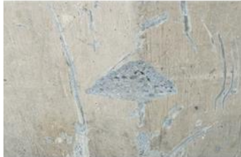
PIER 2 COPING (SPALLING)
