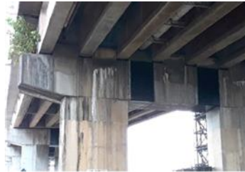
PIER 3 COPING (CRACKING & WATER LEAKAGE; VEGETATION)
