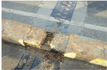
PIER 3 EXPANSION JOINT, SOUTH SIDE (SILTED EXPANSION JOINT; MISSING STEEL PLATE COVER)
