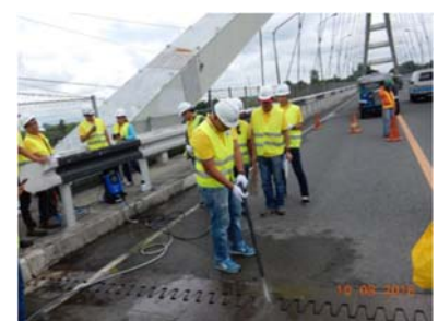
Cleaning of Expansion Joint
