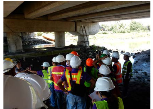
OJT of Bridge Inspection with NDT Equipment (RO-V)
