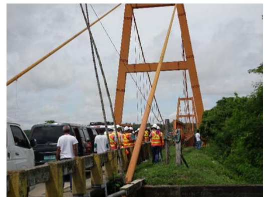
OJT of inspection at Magapit Bridge (Suspension Bridge, RO-II)
